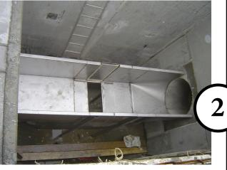
At the bottom of the gutter, there is an opening of precise dimensions
